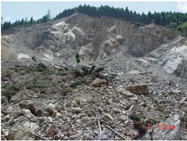
Fig. 1 CAS debris flow
