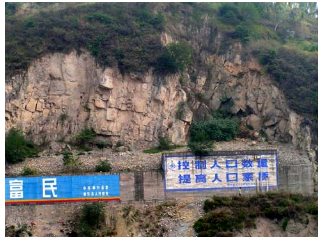
Fig. 6 The outward rotating of the horizontal bedding planes and the toppled blocks (the dash square surrounded area in the Fig. 5)
