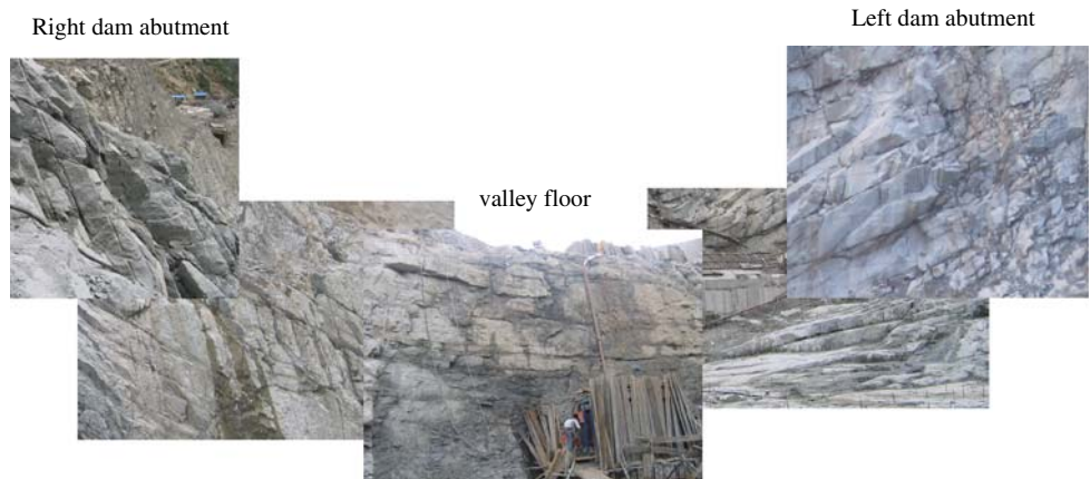
Fig. 5 Unloading fractures caused by stream downcutting in the geological past formed parallel to the morphology of the valley
