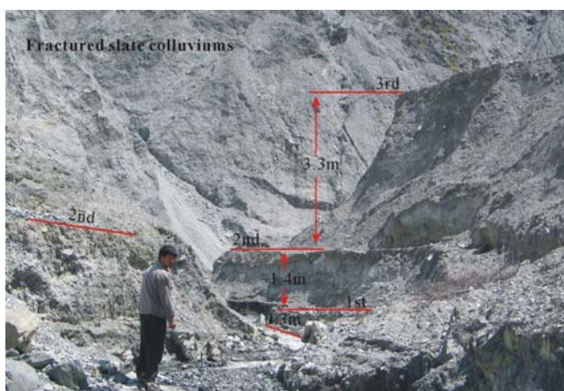
Fig. 9 Site photograph showing fast cutting and severe erosion in Menqian ravine, position (1,660E, 1,280N)
