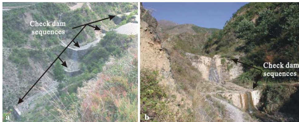
Fig. 4 Site photographs showing sequence of pointed random rubble check-dams in good condition in the debris-flow channels in Duozhao. a Check-dams in Daqishu channel, position (3,240E–2,050N); b check-dams in Dasha channel, position (3,340E–1,310N)
